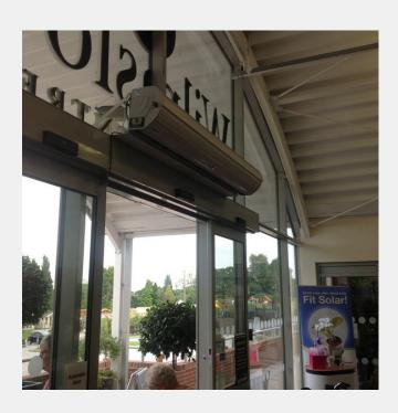
The ingress of any external pollutants, flying insects, odours, and dust were also eliminated making for a cleaner internal environment. As the Enershield Air Barrier draws in ambient air from above, it achieves an element of destratification by bringing hot air down, further reducing heating costs and increasing comfort
